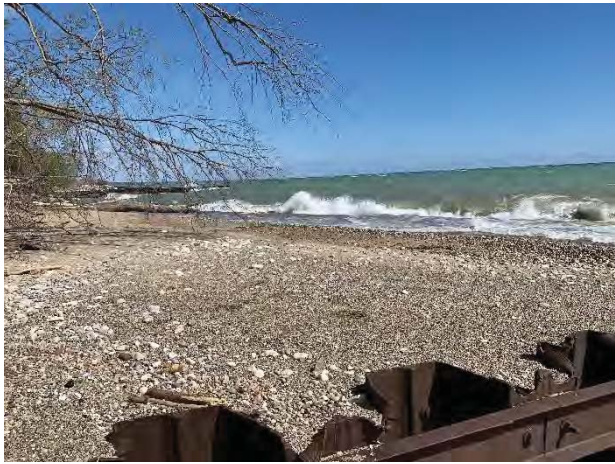
Figure 2.15 Beach front that had been protected due to the existing jetty.
