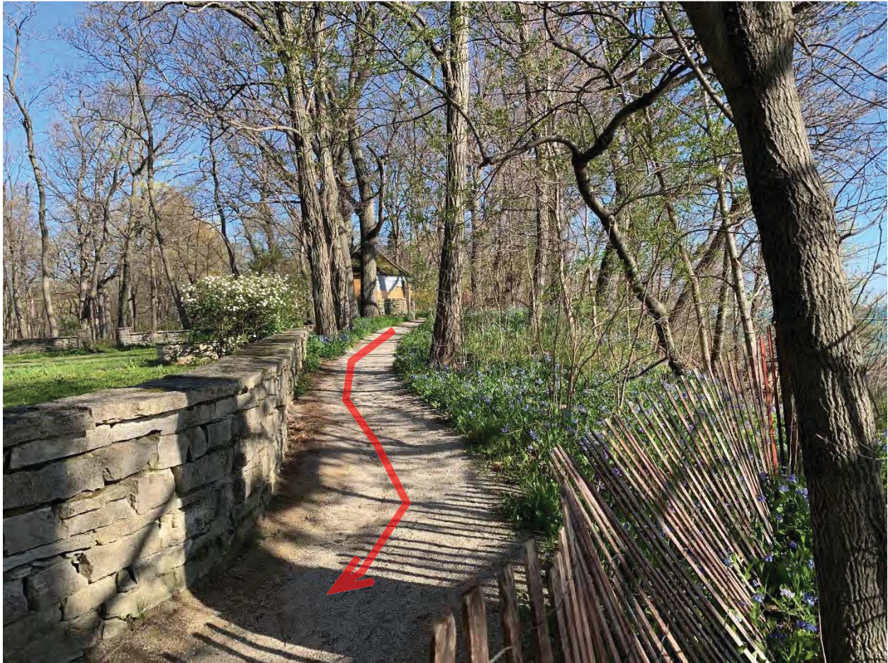
Figure 4.41 Existing top of bluff path being used to focus accumulations of drainage to bluff top edge
