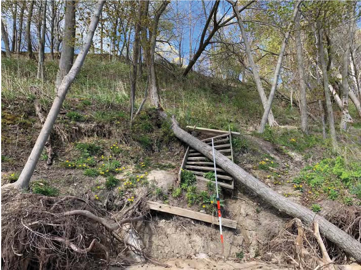
Figure 1.10 Destroyed stair access to beach – also a location expected to fail in the immediate future.
