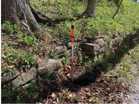
Figure 2.34 Drainage inlet found along Millard Park path.
