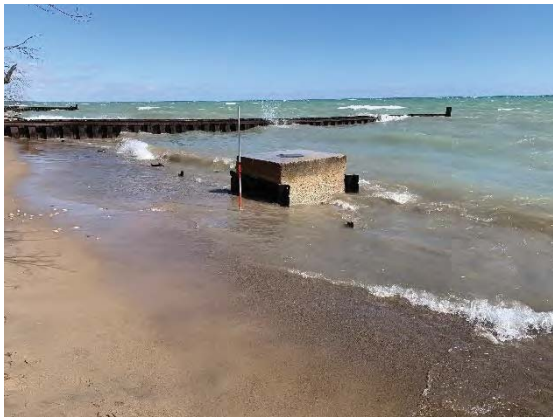
Figure 2.35 Probable MWRD interceptor sewer structure at bottom of bluff.
