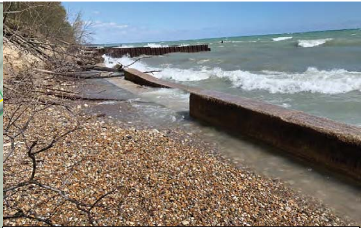
Photo 14: Photo of deteriorating seawall looking north along the beach
