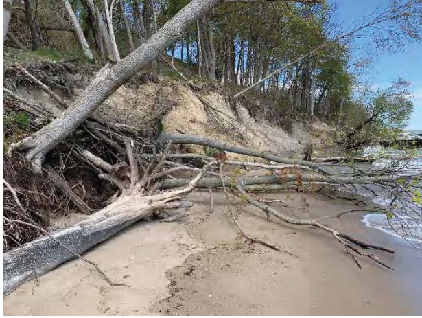
Figure 2.13 Bluff erosion along the beach in Sections A & B.
