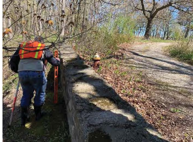
Figure 2.33 Fire hydrant at the northern end of Millard Park on the west side of the bluff.
