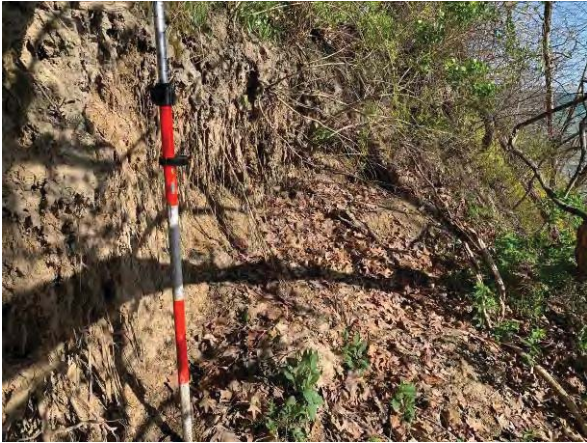
Picture 1: Vertical drop due to slope failure.
