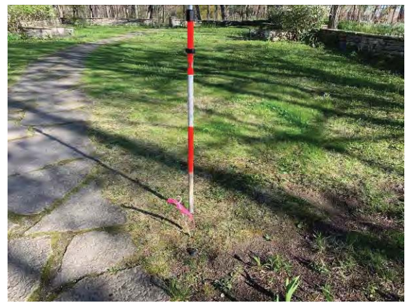
Picture 12: Sprinkler head still in use?
