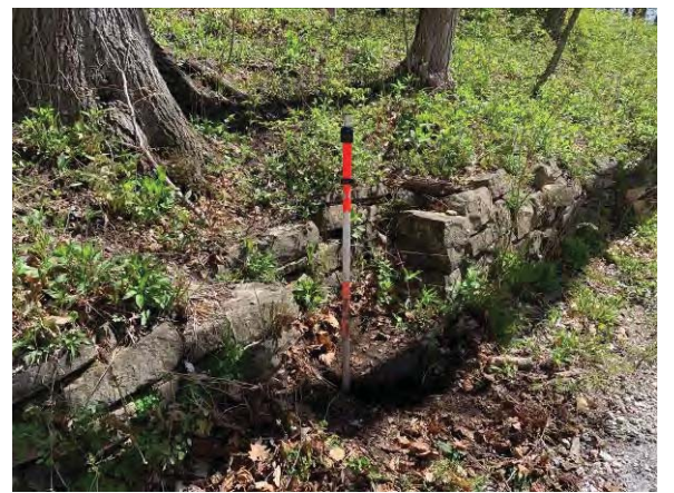
Picture 10: Storm sewer inlet.
