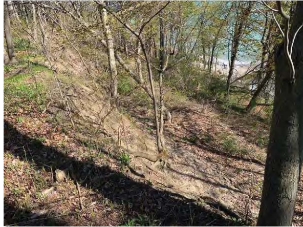
Picture 2: Slope Failure.
