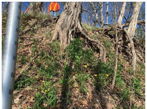
Picture 6: Exposed root system due to erosion.
