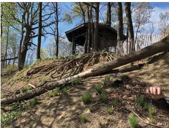
Picture 5: Exposed root system due to erosion.
