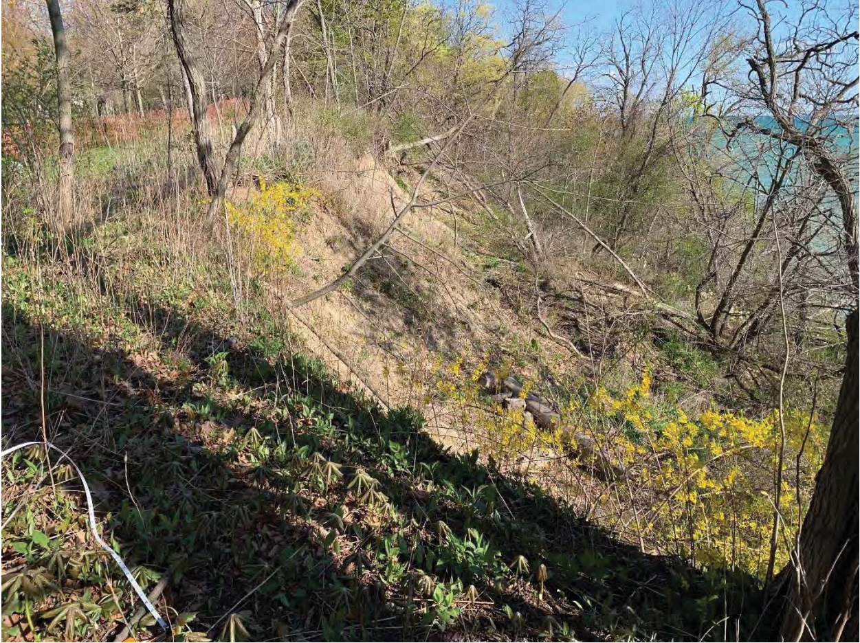
Figure 2.12 Large slope failure in Section B
