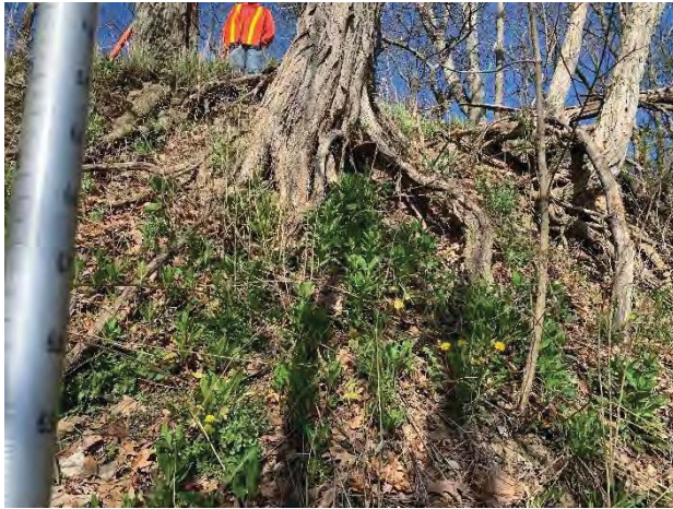
Figure 2.21 Exposed root system due to erosion at north end of Section C.
