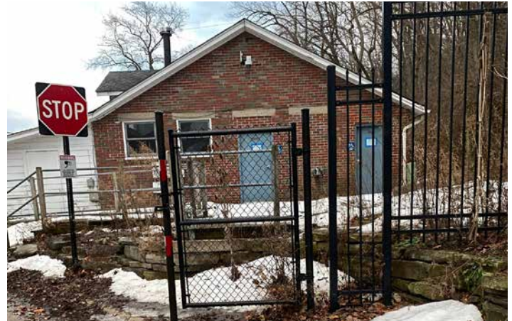
TOP: Existing boat launch conditions at south beach area.
