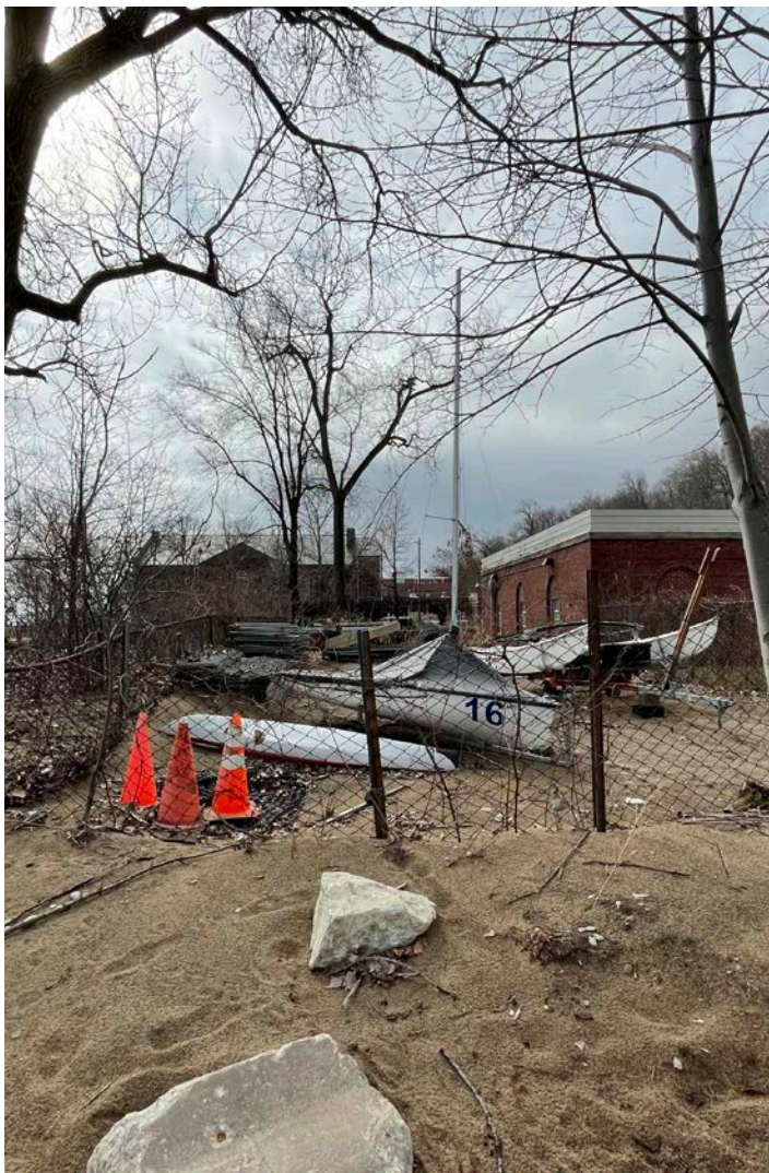
TOP: View of north beach showing exposed protection fabric and migrated shoreline stabilization stones impacting beach area.
