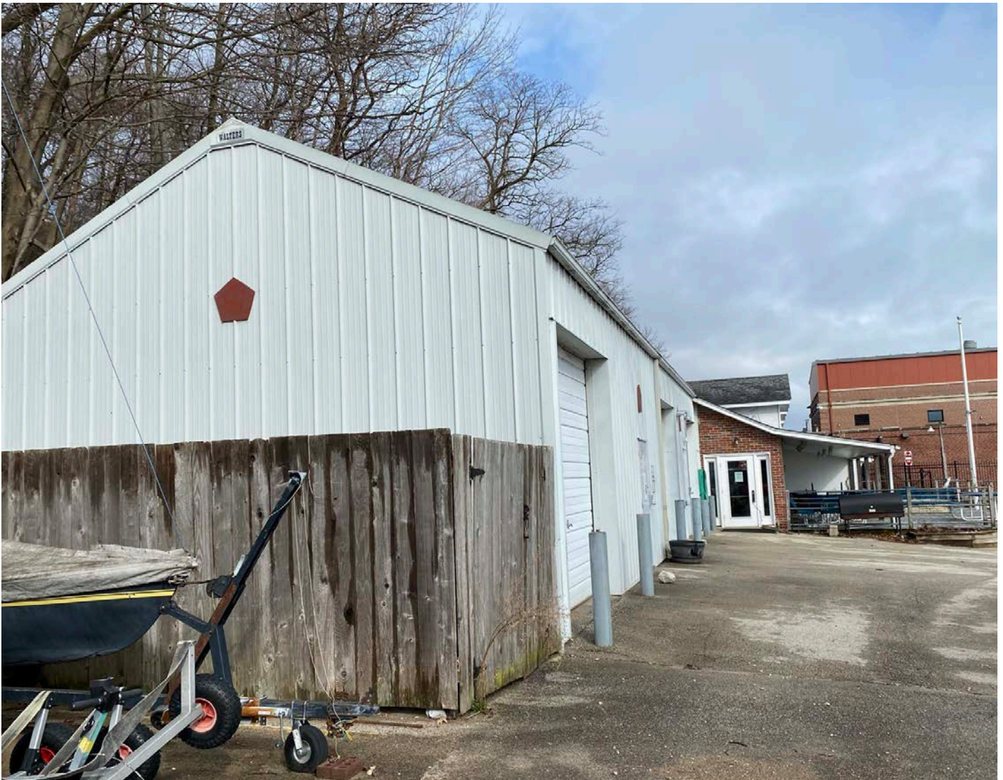
View from vehicle and trailer parking area looking north towards North Shore Yacht Club storage facility.
