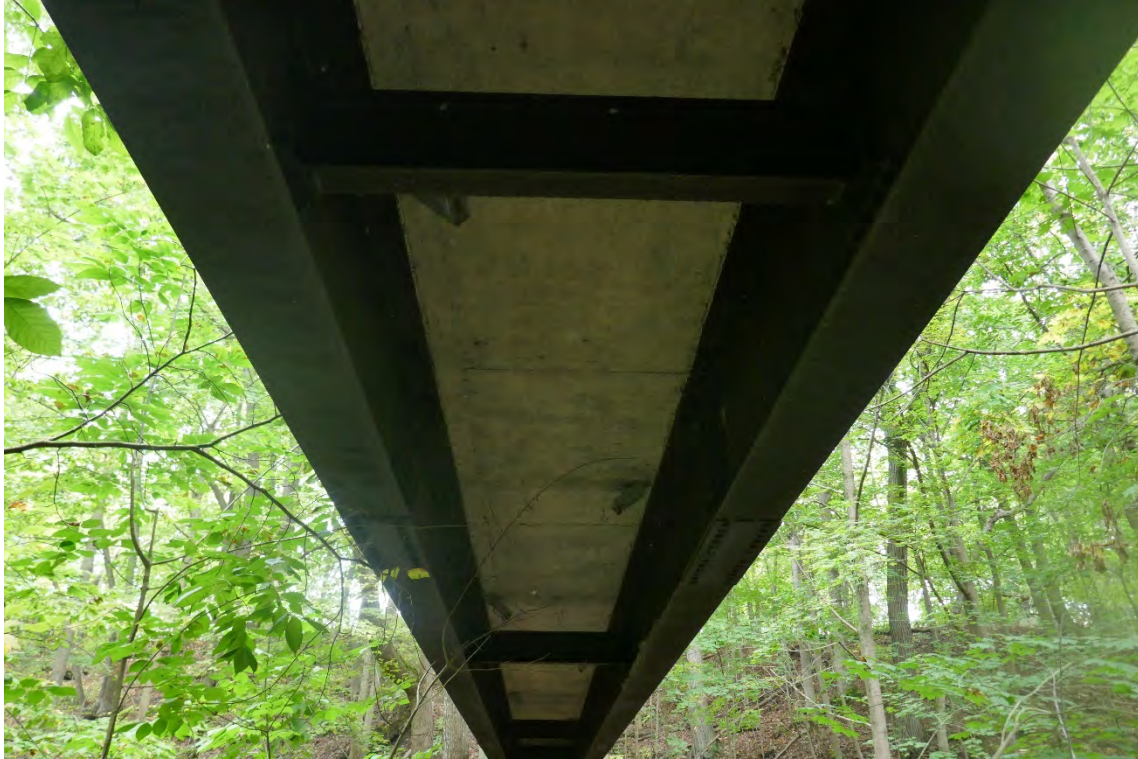
Typical Underside of Deck Condition – Minor Transverse Cracking
