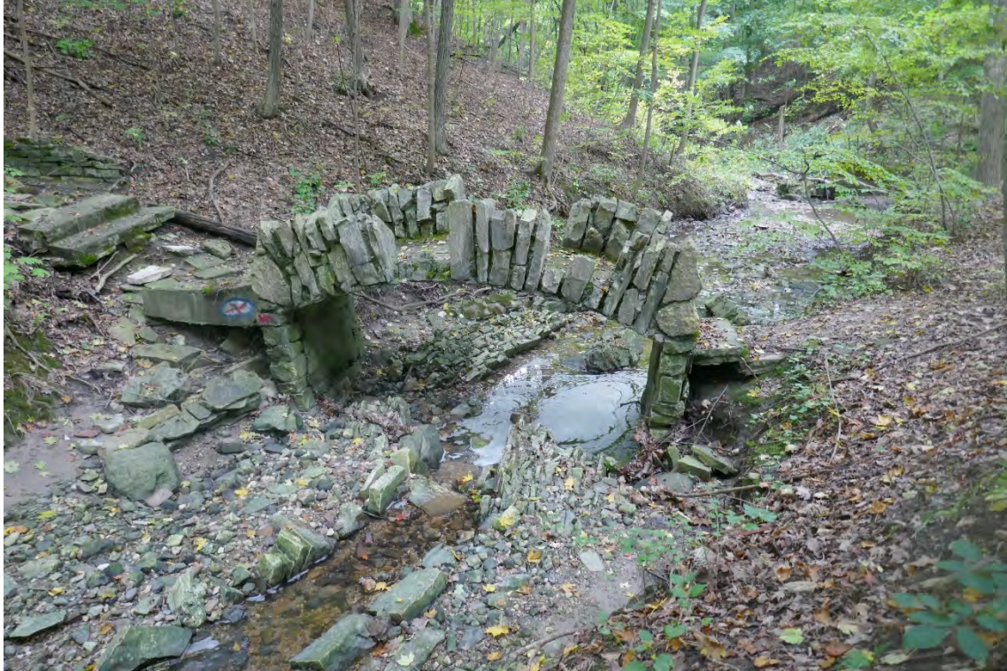
Looking North From Bridge
