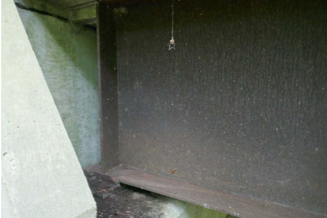
Beam Ends – Good Condition – No Issues Noted
