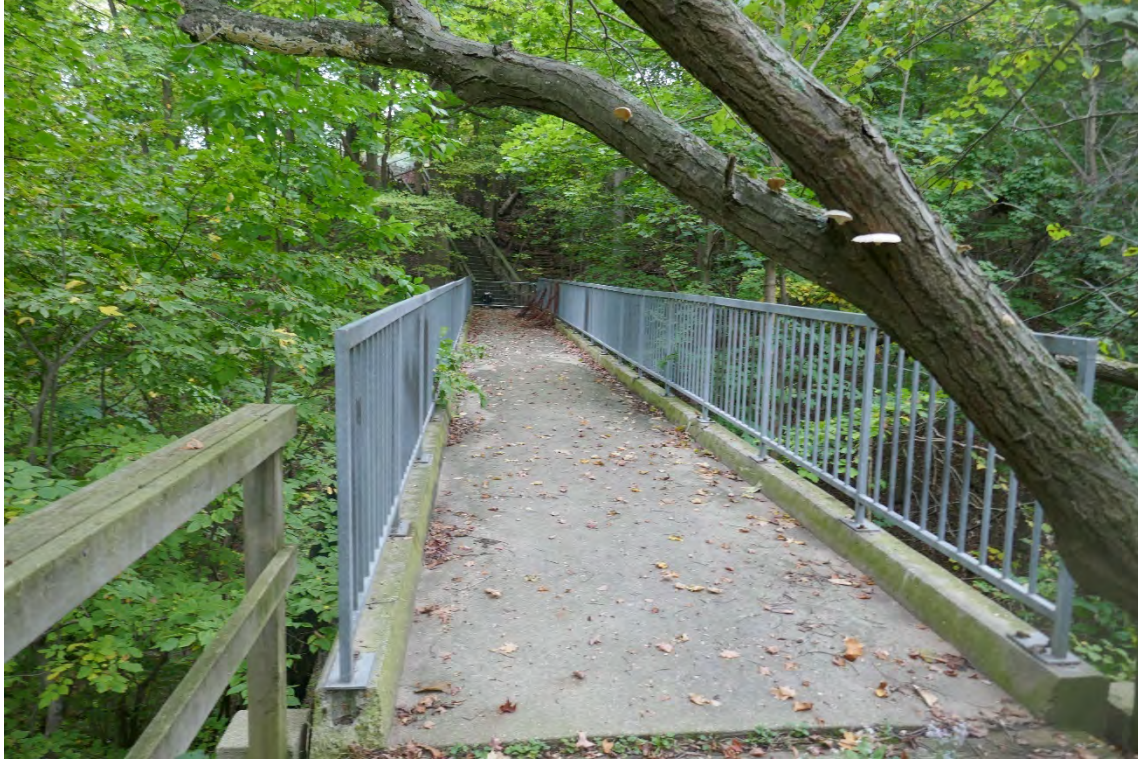
Bridge – Looking West
