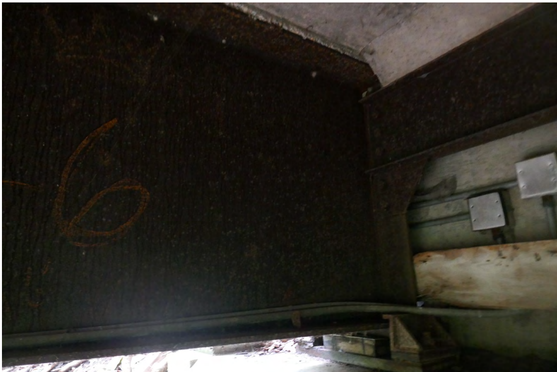
Beam Ends and Bearings– Good Condition – No Issues Noted
