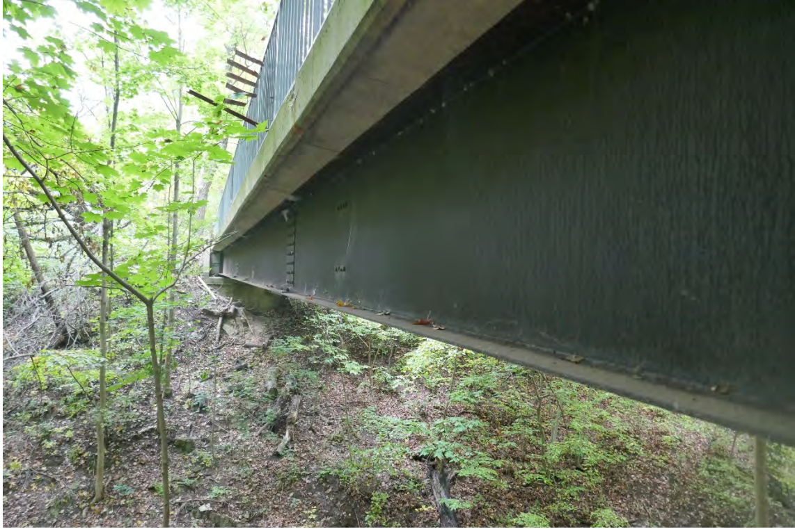
Typical Plate Girder Condition – Good Condition, Including Splices – No Issues Noted
